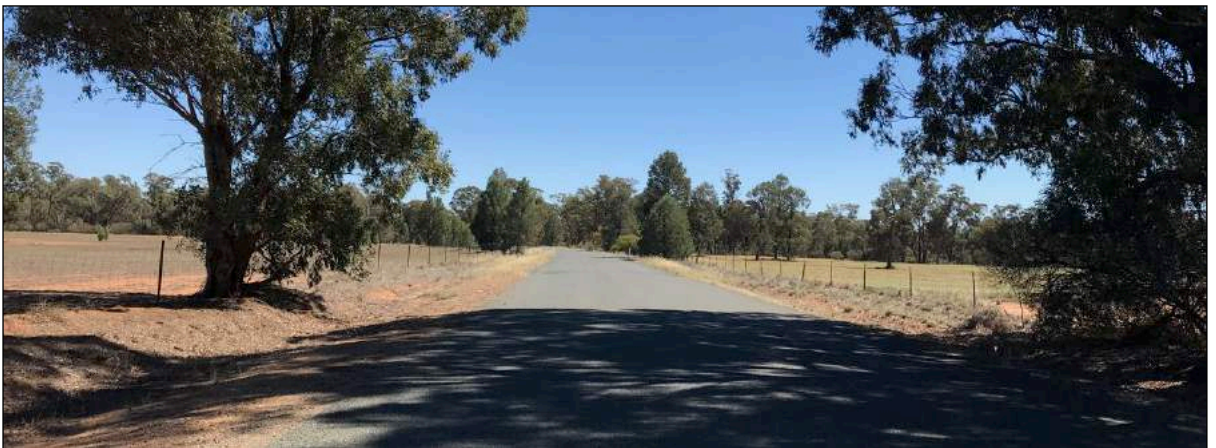
Figure 10: Bellarwi Rd looking N towards creek causeway adjacent Lots 171, 174 & 373 (Source: SP 2018)
