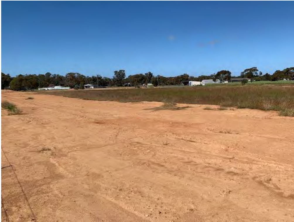
Figure 5: Silt spread around the boundary of the rear paddock.
