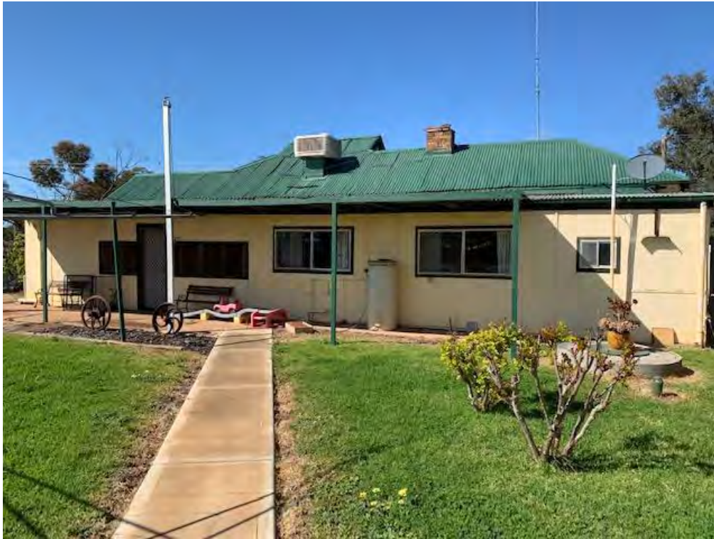
Figure 1: Old smaller house rear extension (potential bonded ACM cladding).
