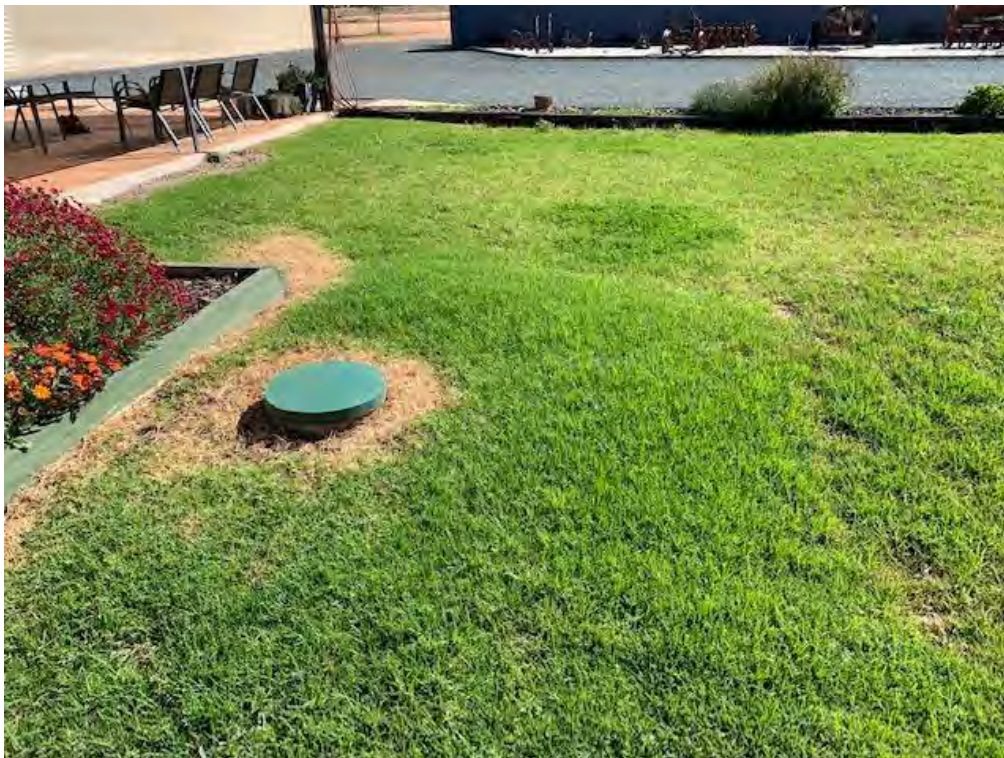
Figure 2: New larger house septic system.
