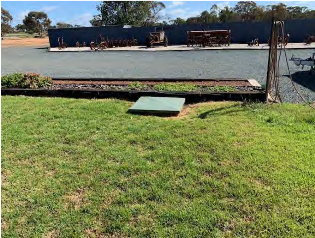
Figure 3: Old smaller house septic system.
