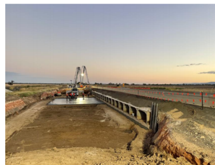
Construction in progress on a new culvert at Murrumbilla Lane in section 1
