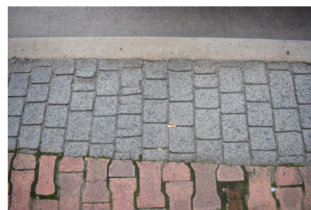
Inconsistent and uneven paving along Main Street requires upgrade
